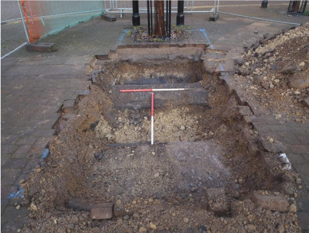
Plate 3. Trench 2, showing services, looking north-west (scales 2m and 1m)
